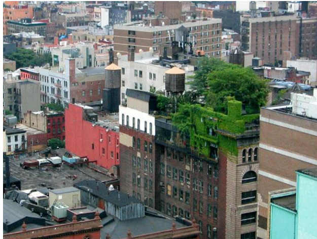
Fig.6 - An intensive roof garden in Manhattan, New York, USA
