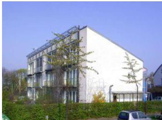
Fig.4 - One of the original Passive Houses at Darmstadt, Germany
